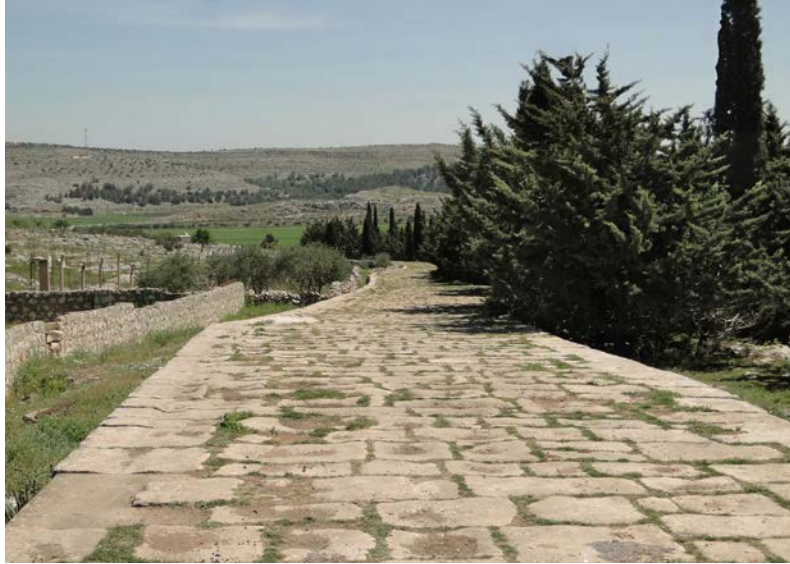
Figure 11.1 - Example of a Roman Roadway Still Maintained
