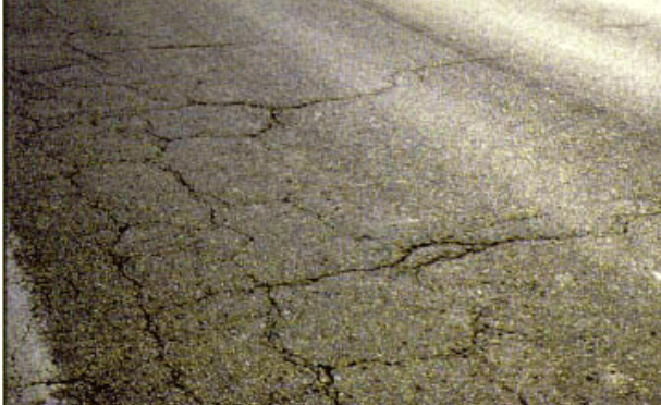
Figure 3.9 - Block Cracking in Asphalt Pavements
