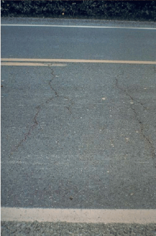
Figure 3.11 - Longitudinal and Transverse Cracking in Asphalt Pavements
