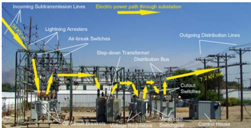
Figure 15.8 -Components of a Typical Substation
