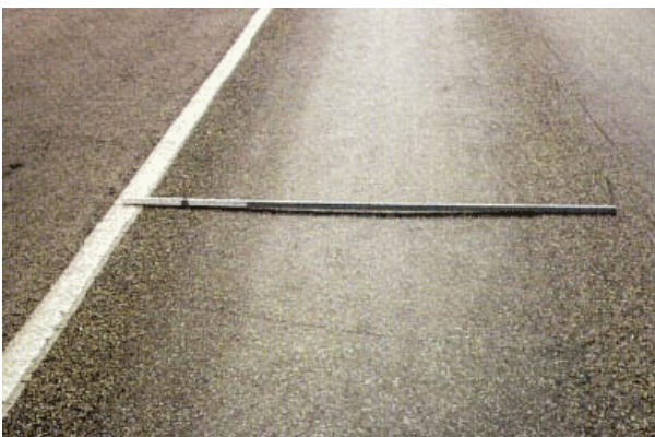
Figure 3.13 - Rutting and Depressions in Asphalt Pavements
